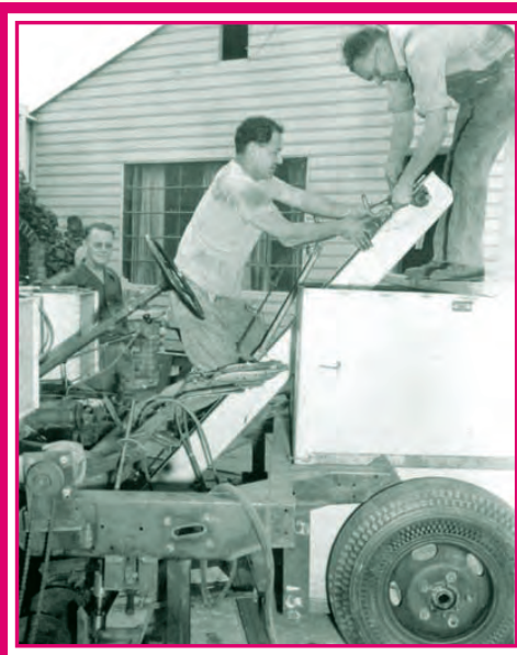
Frank Zamboni building an early prototype of a Zamboni® Ice Resurfacing Machine
