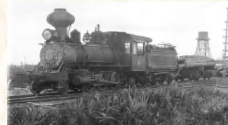
Germain Land and Timber Company log train, 1924, courtesy Tampa-Hillsborough County Public Library System
