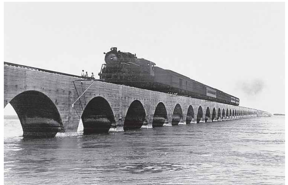
FEC train rumbles over the viaduct of Knights Key Bridge.
