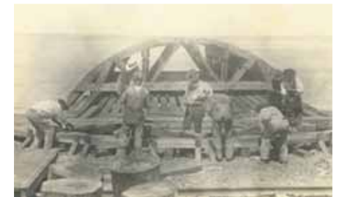
FEC workmen construct part of the Over-Sea Railroad.
