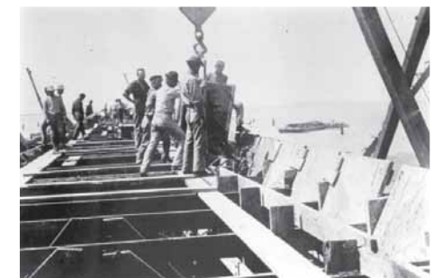
FEC workers construct a bridge on the Over-Sea Railroad. (State Archives of Florida)
