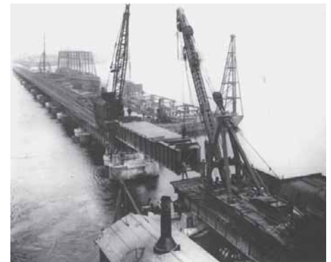
Construction of double bridge in Jacksonville. (State Archives of Florida)
