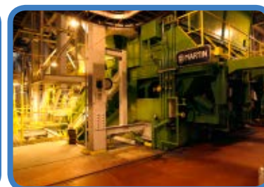
At the Hillsborough County Resource Recovery Facility, huge furnaces burn municipal waste to produce electricity. Skip O'Rourke, Times file photo
