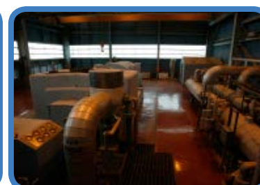
Steam produced from the burning of municipal waste turns a turbine to power a generator that produces electricity at the Hillsborough County Resource Recovery Facility. Skip O'Rourke, Times file photo
