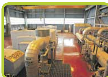
Steam produced from the burning of municipal waste turns a turbine to power a generator that produces electricity.
