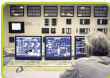
Workers monitor all systems in a control room deep inside the plant and control the production of electrical power from municipal waste.
