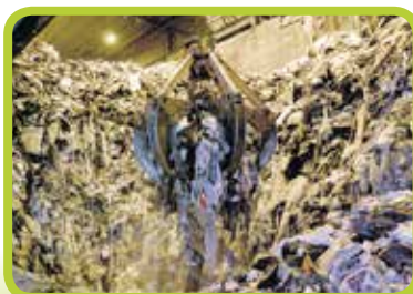
Garbage is lifted by crane and placed into a hopper.
