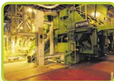
Huge furnaces burn municipal waste to produce electricity.
